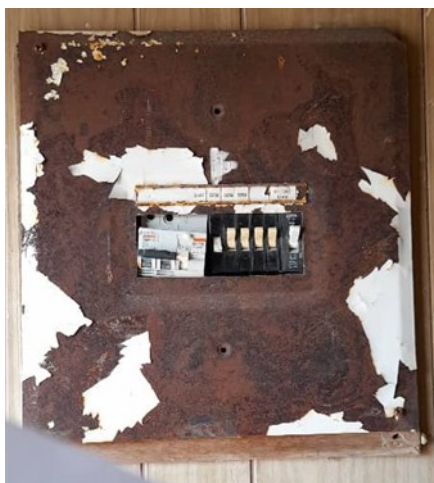
Distribution panel in the office cabin corroded and incorrectly labelled
