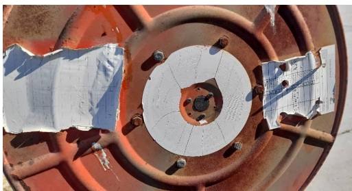
Fire hose reels are old and have no record of inspection
