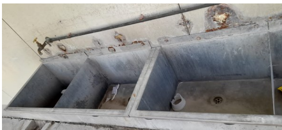
Taps missing on Washing Basins
