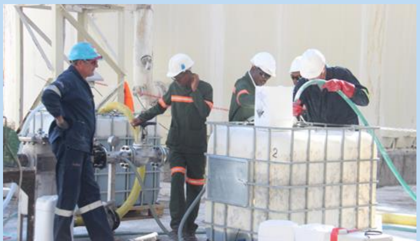
Shell and heat plate exchanger chemical cleaning at the carbonation plant- Soda Ash (File Pic)
