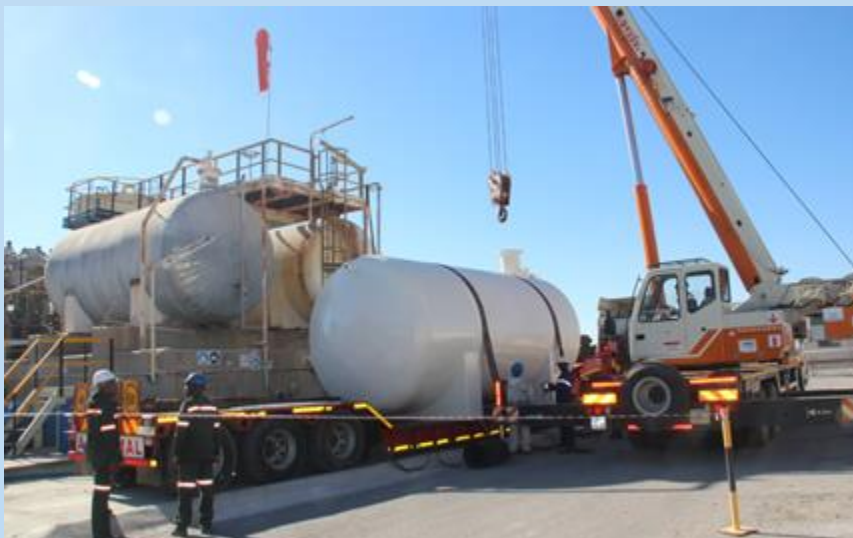
A crane lifting the sulphuric acid tank at carbonation plant in preparation for replacement. (File Pic)
