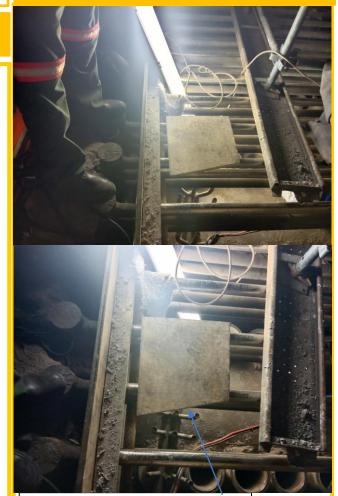
Shutter board used for providing walking platform on the boiler tubes
