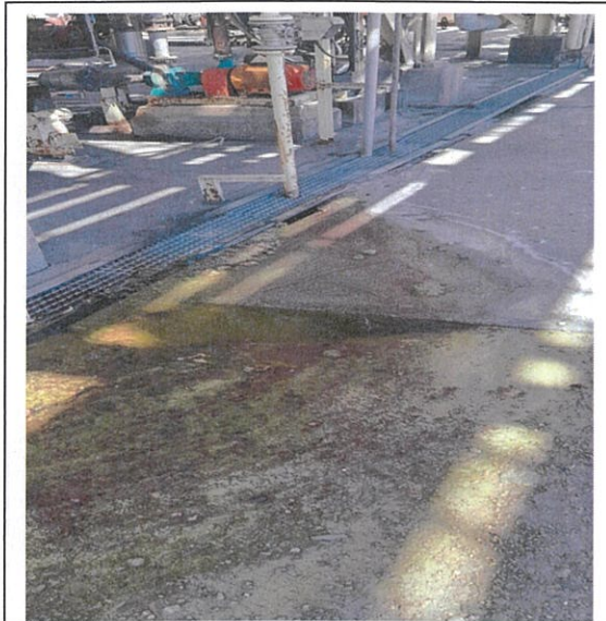
Underground Pipe Leak
