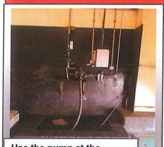
Use the pump at the vehicle workshop to decant oil into the used oil
