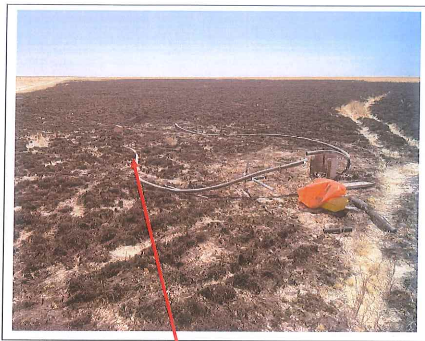
Exposed electric cable
